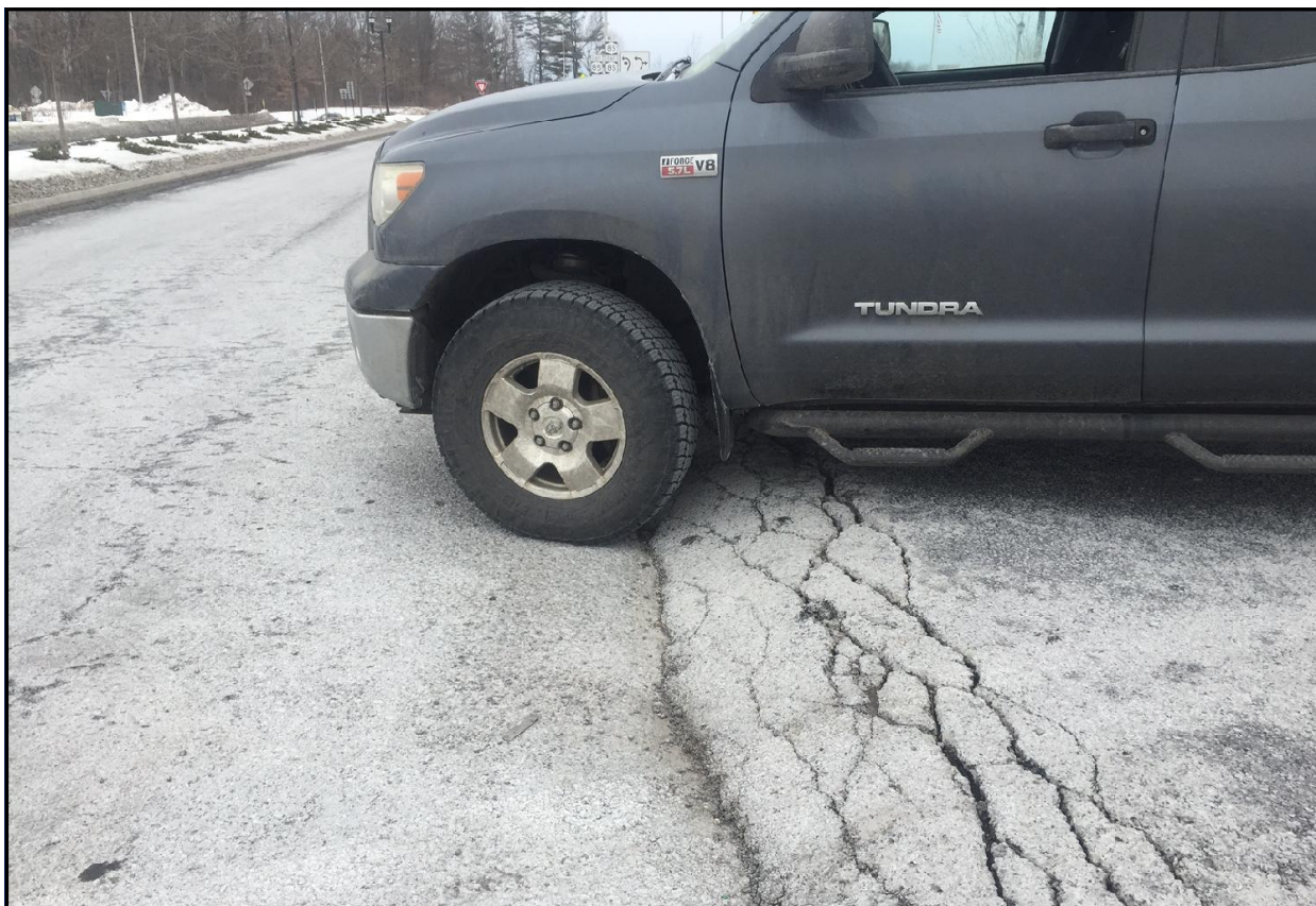
Frost Heave - 03/05/ 2015 – Project Specifics Unknown
