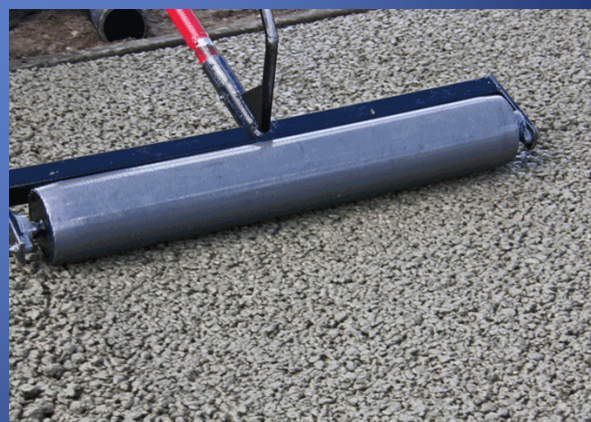
Poured in Place Porous Concrete
