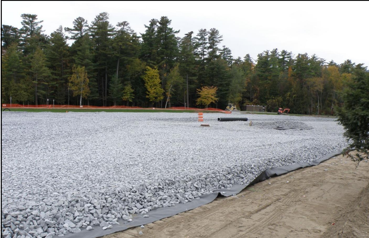
NYSDEC - $M Beach Reservoir Stone beneath both Porous & Conventional Pavement – October 2014
