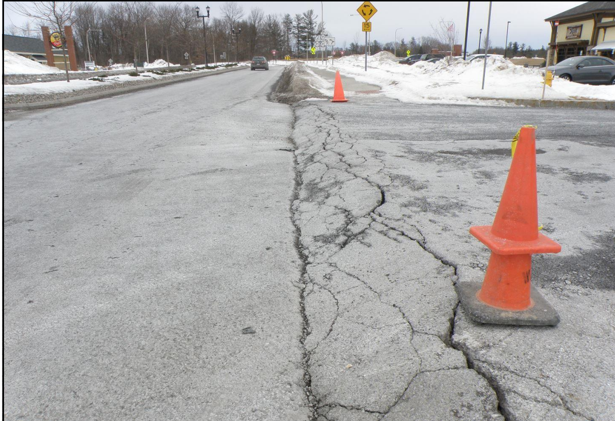
Frost Heave - 03/05/ 2015 – Project Specifics Unknown
